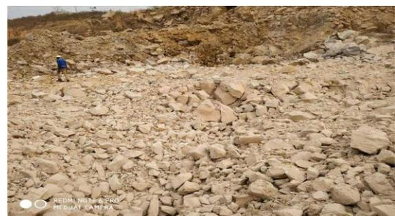
**Figure 5:** Field Photograph Showing Blasted Rocks with the Recommended Parameters.
