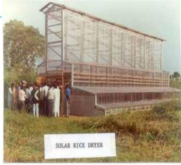
2-tonne Solar Rice Dryer at Adarice Co. Enugu built by NCERD
