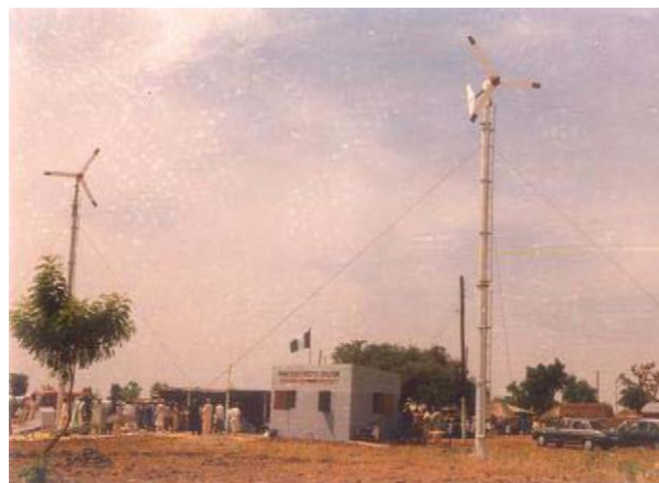
Figure 6: 5 kW Wind Power for Village Electrification, Sayya Gidan Gada, Sokoto State Built by SERC.
