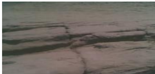
Figure 13: Joint Observed on Awe Formation.
