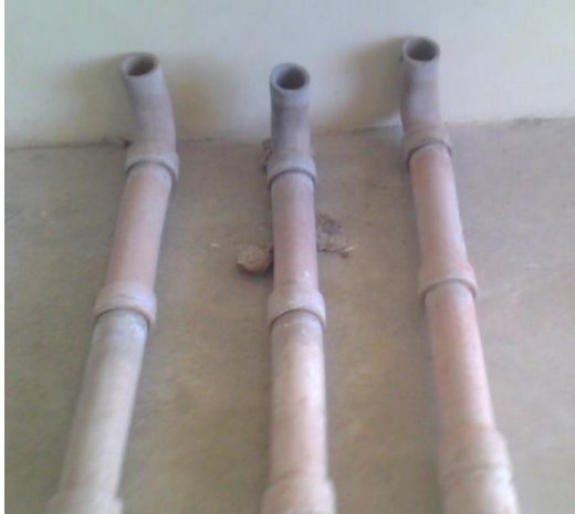
Plate 3: The assembled clay pipes.
