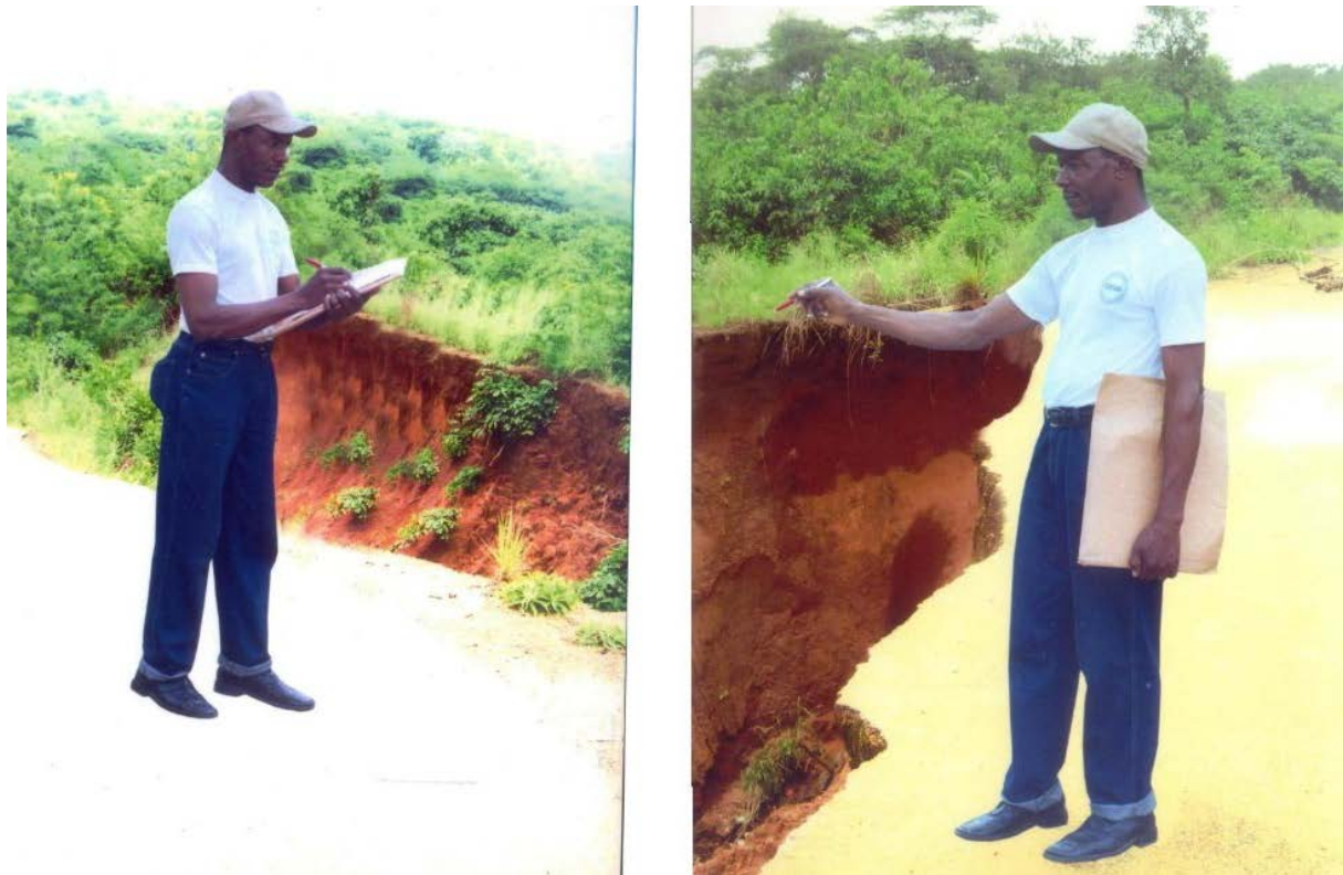
Figure 10: Deep Gullies Located Near ABSU.
