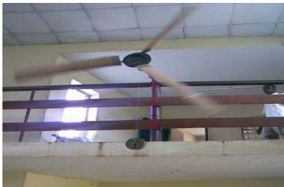
Figure 2: Turbine Mounted on the Gantry.
