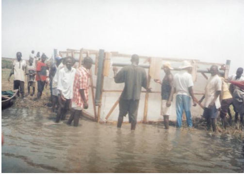
Figure 5: Transporting the Cage to the Dam.
