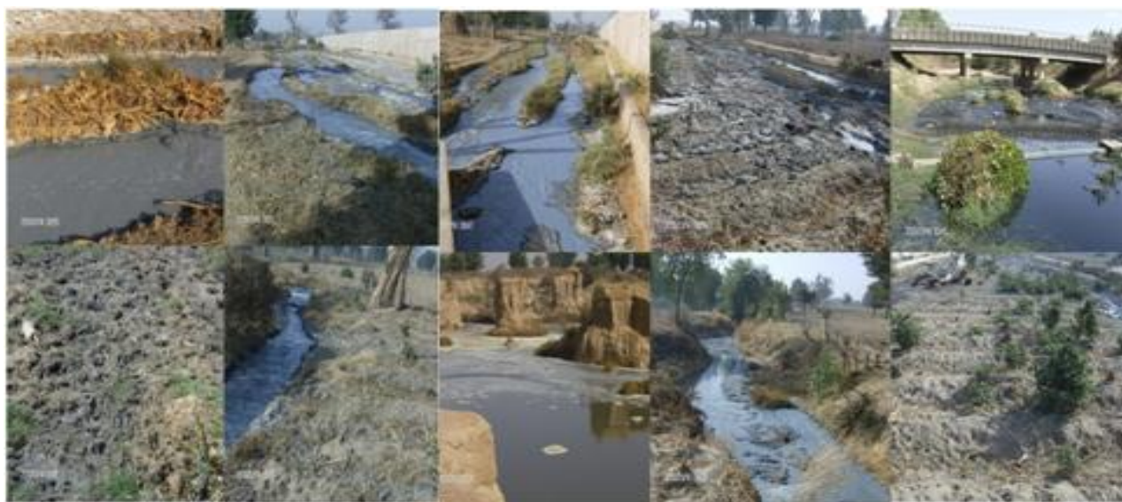
Figure 2: Photographs Showing Some Effluent Channels and Some Contaminated Farm Lands between the Challawa Industrial Site and the River Challawa .
