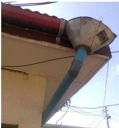
Figure 4: The Funnel and the PVC Pipe Conveying the Water to the Storage Tank Viewed from a Different Angle.
